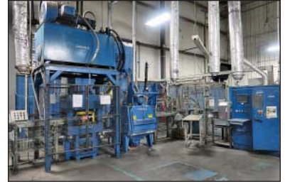
(5) Shop Fabricated Coining Press Lines w/ Presses and Hydraulic Units, Blasters, Robots, Control Panel and Electrics
