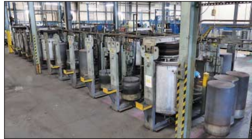
Shop Fabricated 24-Station Electric Bell Furnace with 5 Heating Kettles
