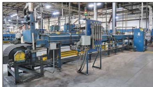
(2) 24" x 65' General Electric 40XGO2267G1 Mesh Belt Continuous Electric Furnace
