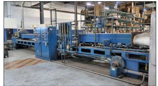
(4) Belt Furnaces and (4) Bell Furnace Systems
