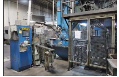
(9) Shop Fabricated Up-Acting Hoop/Mold Presses with 36", 16" and 12" Rams
